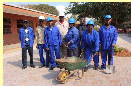
Mokopane bricklaying team after completion of paving at Sekgooa Kgala Lower Primary School Mahwelereng
